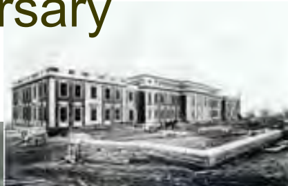
Building 307 under construction
